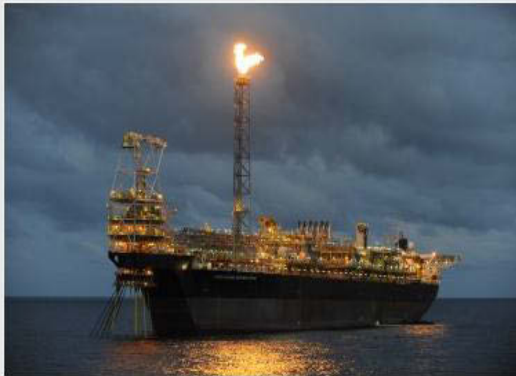
The Kwame Nkrumah Floating Production, Storage and Offloading facility in Ghana's offshore Jubilee Field, operated by Tullow and partners. (Photo: Tom Fowler)
